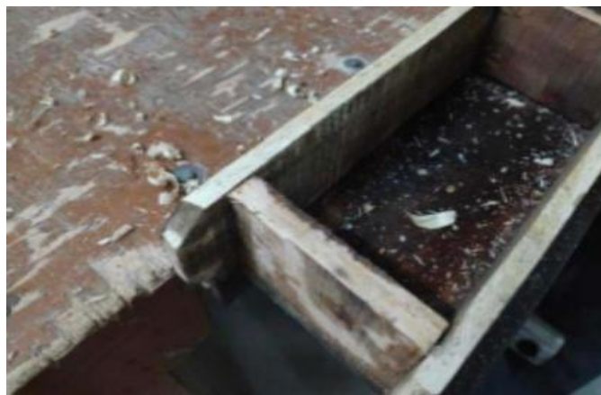
Fig.1: Preparation of mould in carpentry shop
